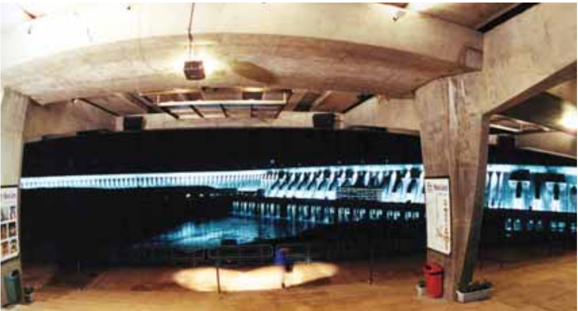
The Itaipu hydroelectric plant and dam [shown] was one of the stops on a three-day tour of different facilities in southern Brazil organized by the IEEE student branch at the Universidade Estadual Paulista in Bauru, Brazil.
