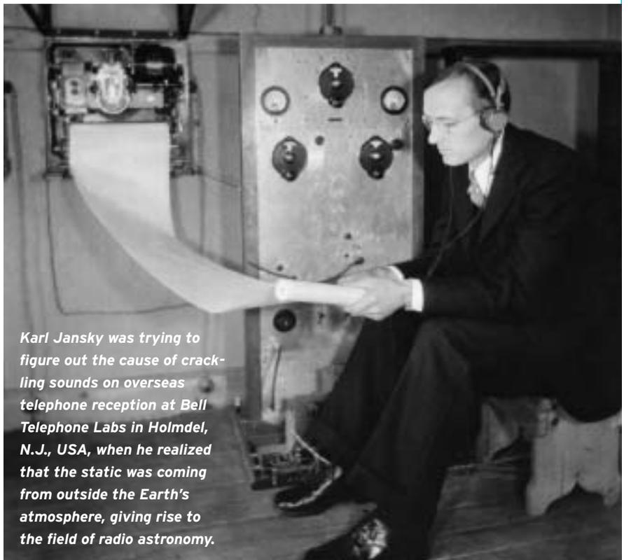
**Karl Jansky was trying to figure out the cause of crackling sounds on overseas telephone reception at Bell Telephone Labs in Holmdel, N.J., USA, when he realized that the static was coming from outside the Earth's atmosphere, giving rise to the field of radio astronomy.**
